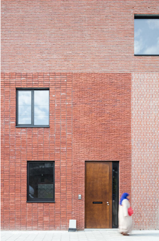
Figure 18: PTA109 . Apartment building, Antwerp (fotos Tim Van De Velde)
